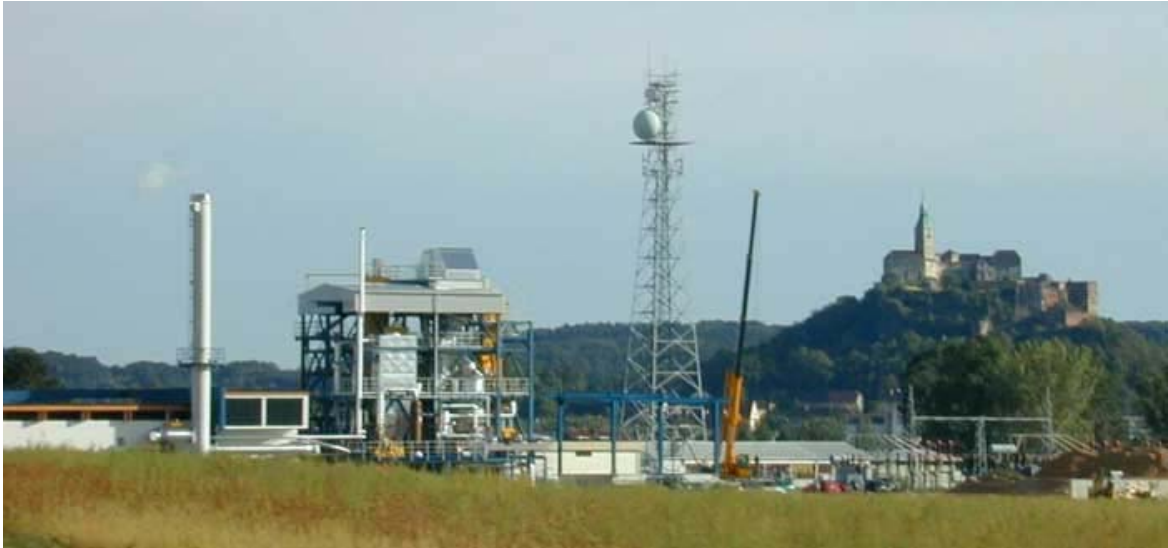
Figure 1 2 MW el /8MW th biomass CHP plant in Güssing (Source: RENET Austria)
